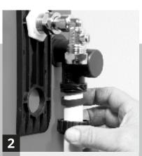
Connect overflow to Compression Warning Pipe assembly ensuring warning pipe accommodates incoming supply.
