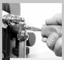
Turn on the Cold water Supply (stop cock usually under the sink) Then turn the Service Valve using a screwdriver to the on position(in line with the water flow). As the tank fills check all round for leaks with Hand and Eye. Clip Down the Lid.
