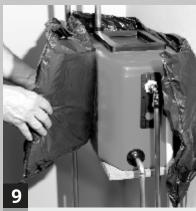
Fit the Insulation around the Polytank.
