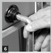
Connect outlet into Push Fit Tank Connector. This Tank Connector accommodates 15mm Pipe.
