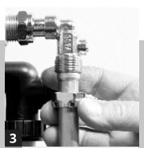
Connect incoming Cold Feed into the Compression Angled Service Valve. This angled Service Valve accommodates 15mm Pipe.
