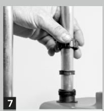
Remove Expansion Pipe Nut and Washer and fit 22mm Expansion Pipe though the Expansion Pipe Sleeve. Replace Nut and Washer and Tighten.
