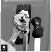
Ensure the other end of the Angled Service Valve is Nipped up securely onto the Ballvalve Thread.
