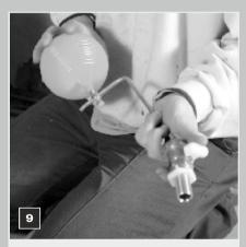
Take your ball valve attach the 41/2" float and assemble into the tank.
