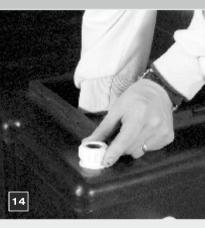
Fit the screwed vent pipe sleeve for the expansion pipe.
