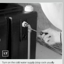
under the kitchen sink) and then turn the service valve using a screw driver, to the on position (in line with water flow).
