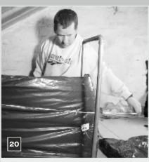
Fasten the insulation using the ribbon provided.
