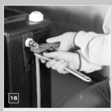
Attach the cold water pipe (inlet) to the service valve connection and tighten ensuring fittings are held firm while tightening. DO NOT OVER TIGHTEN.
