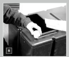
Offer up and mark holes for the breather and vent using a sharp 27mm hole saw, drill the holes for the breather and the vent. All the drilling and marking of the holes can be done at a lower level than the roof space. Once drilled, the tank can be passed up through the loft opening prior to the fitting of any of the kit.
