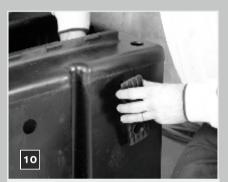
Pass the brass connector through and attach the ball valve back plate to the outside face of the tank. This back plate is designed to spread the load of the continually moving ball valve as the tank empties and fills. Assemble service valve onto ball valve. Adjust float position to suit waterline in tank.
