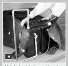
Add the insulation jacket that was provided with the tank kit, wrapping the larger section all the way round the tank.
