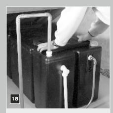
As the tank fills, check all round for leaks both with eye and hand. Clip down the lid/s.
