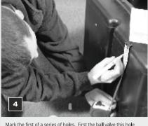
Mark the first of a series of holes. First the ball valve this hole is situated 60mm (+/- 5mm) from the top of the tank. Mark the hole to be drilled with a light marker or crayon. Do not use any scribe or sharp instrument whatsoever. Make a mark for the warning pipe hole - this should be 90mm (+/- 5mm) from the top using a sharp 22mm hole saw, drill the hole for the ball valve and 27mm hole saw for the warning pipe.
